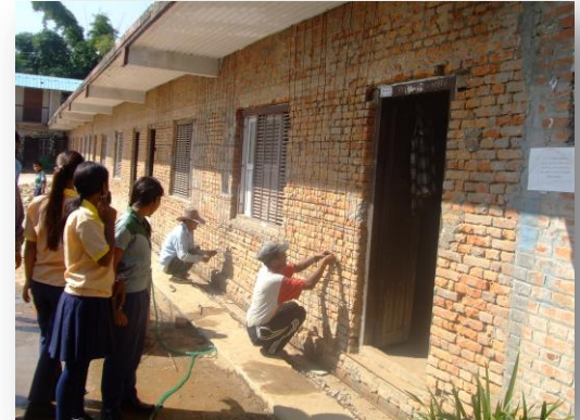
A public school is being retrofitted under the School Safety Program
